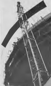
HIGHER AND a little to the right... Fitting large tank plates in place requires effort similar to decking a ship. Coordination between guide, crane operator and workers on tank is on a split-second basis. MAS HALTO y poco pa drechi... Ponemento di plachina grandi di tanki na nan lugar ta exigi esfuerzonan similar cu pa drenta un bapor na waf.
